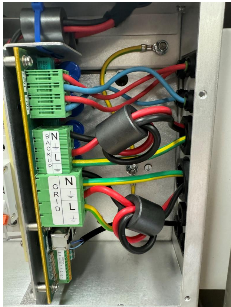
Figure 16 - Grid and Backup Connections
